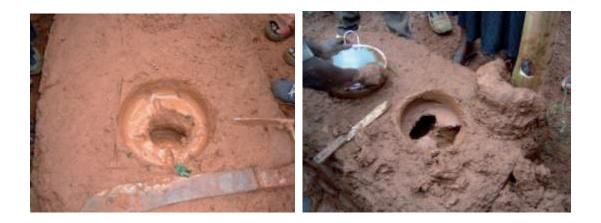
Wrap some of the potato vines with the mixture to form the chimney. Shape as required.
