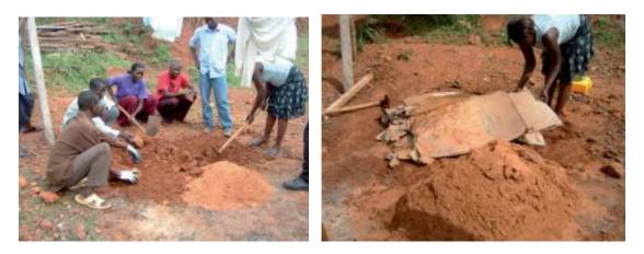
Take off leaves from potato vines and mash in water. Sieve the mixture of sand and soil. Mix this water into the soil/sand mixture – trample it in with your feet, so that it is all thoroughly mixed well together.
