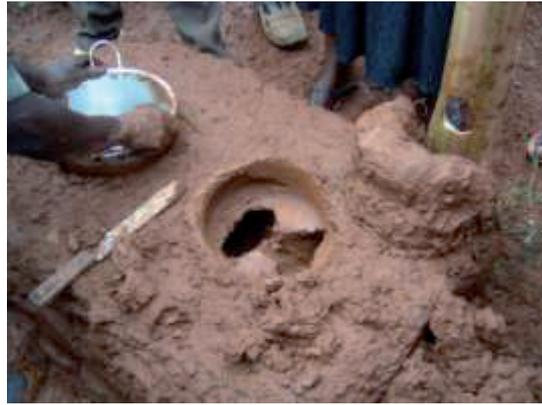
Wrap some of the potato vines with the mixture to form the chimney. Shape as required.
