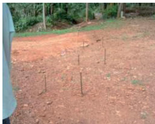
Do 2 rows. Build your trench diagonally from the first marker of the first row to the second marker of the second row.
